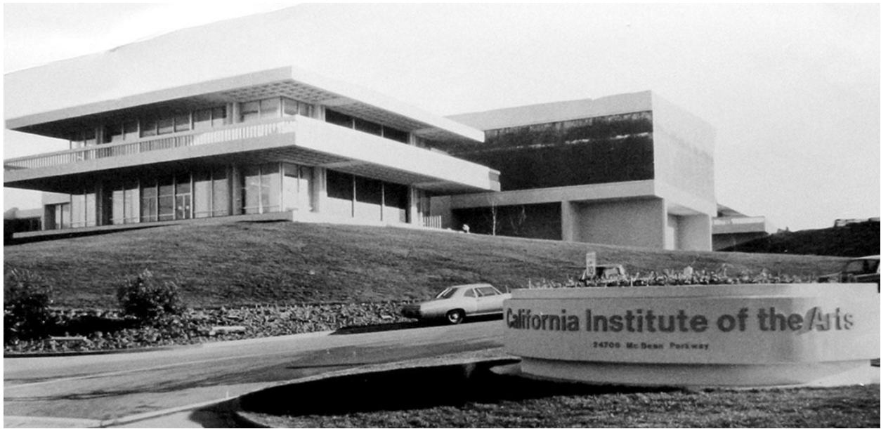
CalArts building designed by firm Ladd & Kelsey, 1972. Photograph courtesy of East of Borneo
